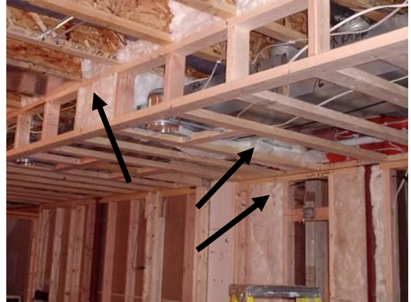
6. Fiberglass insulation used as fire-blocking every 10 feet horizontally in the soffit and separating soffit from wall cavity.
