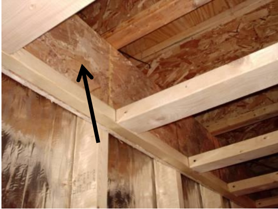
5. Plywood used as fire-blocking from the soffit to the wall cavities.
